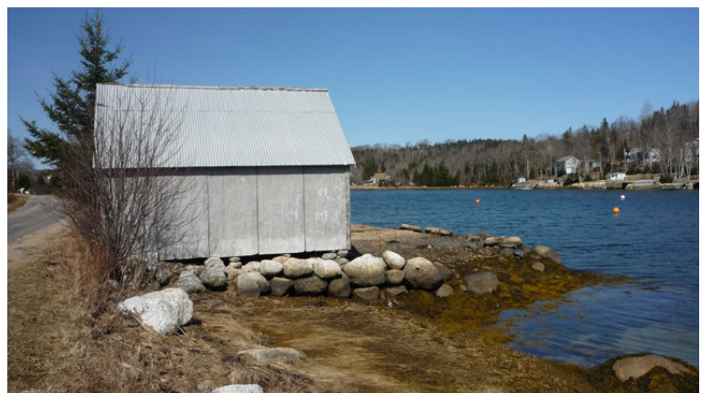
Figure 23: eroding coastline and threatened building, Marriot's Cove Road West.
