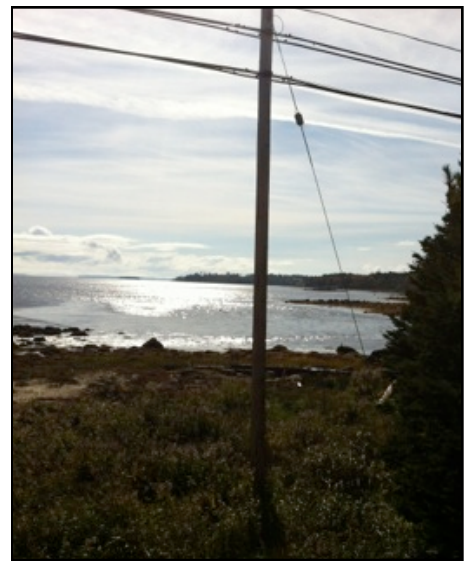
Figure 3: Image, taken from Hwy 3, of a power pole located on the south side of the road. © B. Howard 2011
