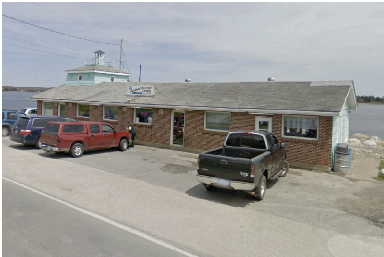
Figure 9. A picture showing the Island View Family Restaurant and Bakery (green canteen) and its proximity to the shore. Photo: Google Street View.
