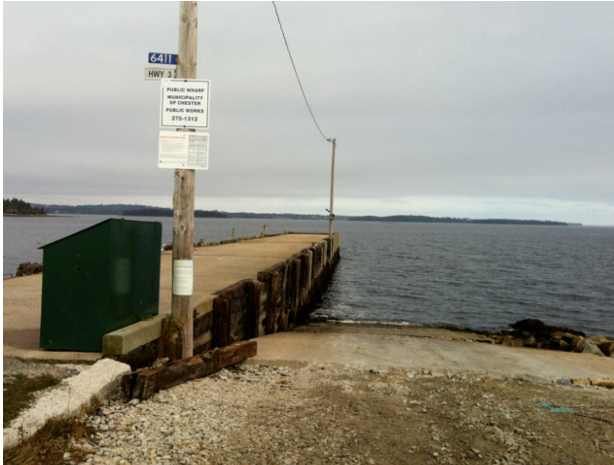
Figure 11. A photograph of the public wharf located on the Western Shore. Photo: Jana Aker.
