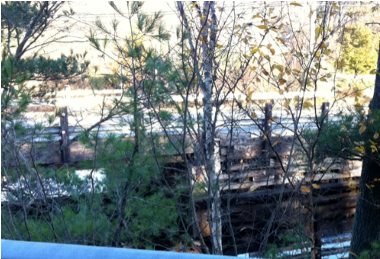
Figure 13. An image showing the proximity of Martins River Bridge to the water. Photo: Jana Aker.
