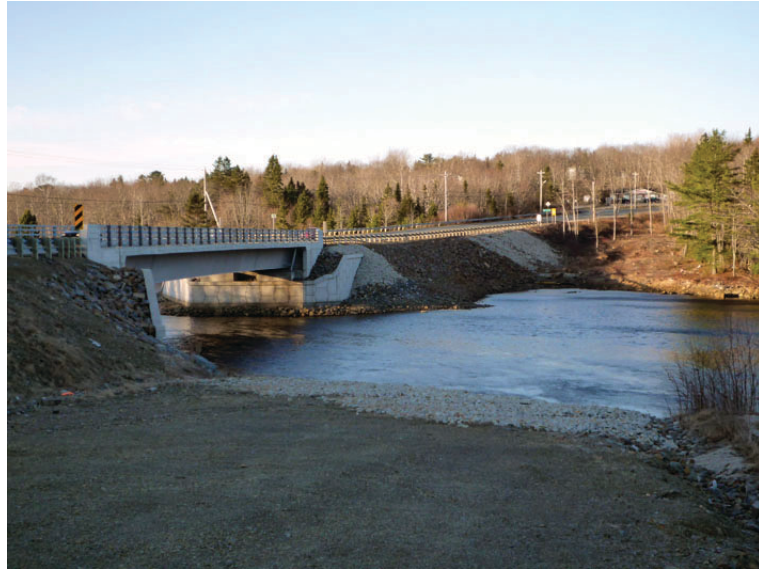
Figure 44: newer bridge at Gold River.
