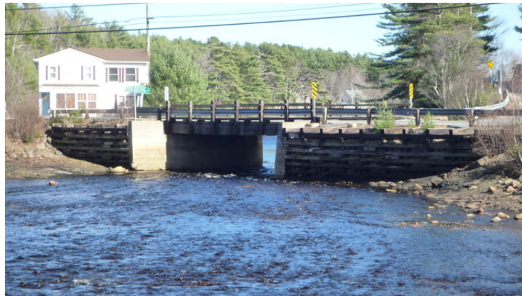
Figure 2: Trunk 3 bridge at Martin's River.
