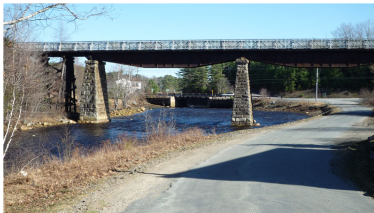
Figure 45: former railway bridge at Martin's River (foreground) with Trunk 3 bridge in the background.
