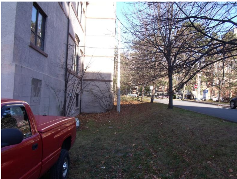
Land sloping toward building. A cistern/planter box will be installed here.
