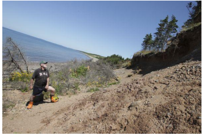
Jim Guy looks over the erosion along the bank of his cottage property in Long Point, near Judique, on Monday. Steve Wadden - Cape Breton Post
