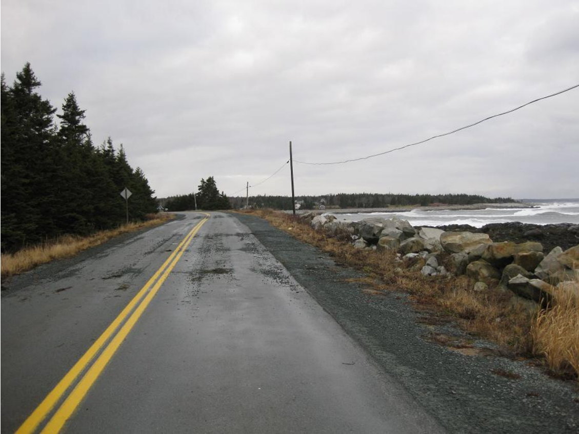
Figure 21 Western Head after Dec 6, 2010 storm surge. Nail in power pole marking the high-water elevation. Note the gravel from the beach deposited on the road.
