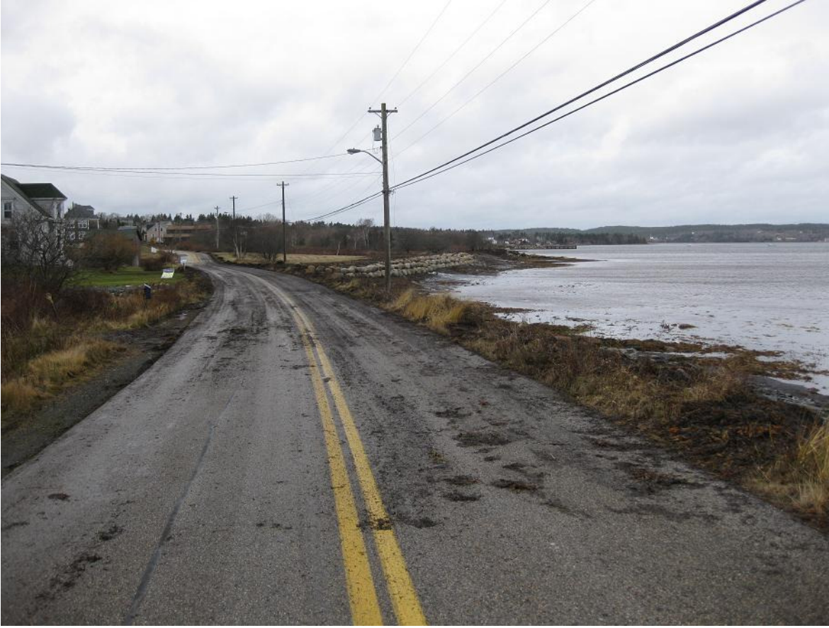
Figure 19 Kingsburg Road Cove after Dec 6, 2010 storm surge. Nail in power pole marking the high-water elevation. Note the gravel and debris from the beach deposited on the road.
