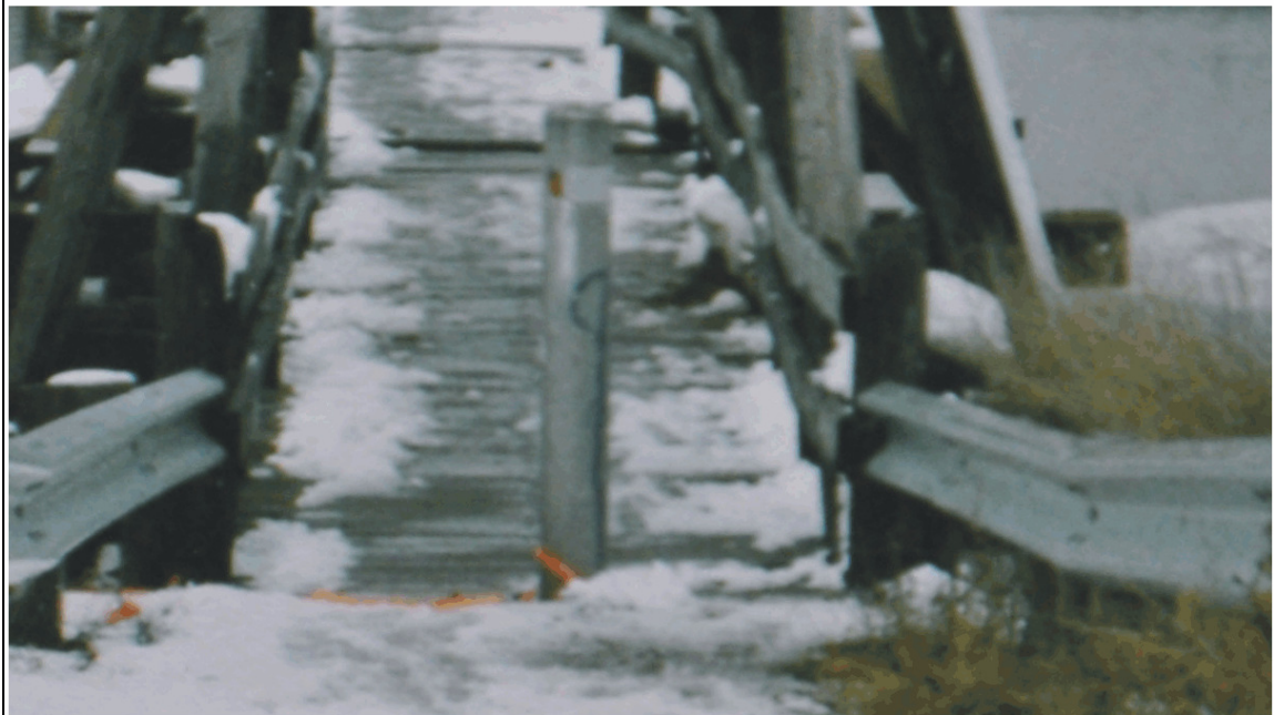
Figure 7 Foot bridge in Port Elgin covered in water during the storm surge event Jan 2, 2010 (top) and after the storm (bottom).
