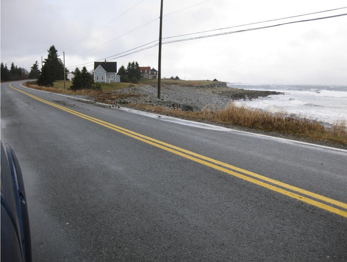
Figure 17 Broad Cove after Dec 6, 2010 storm surge. Nail in power pole marking the high-water elevation. Note the gravel from the beach deposited on the road.
