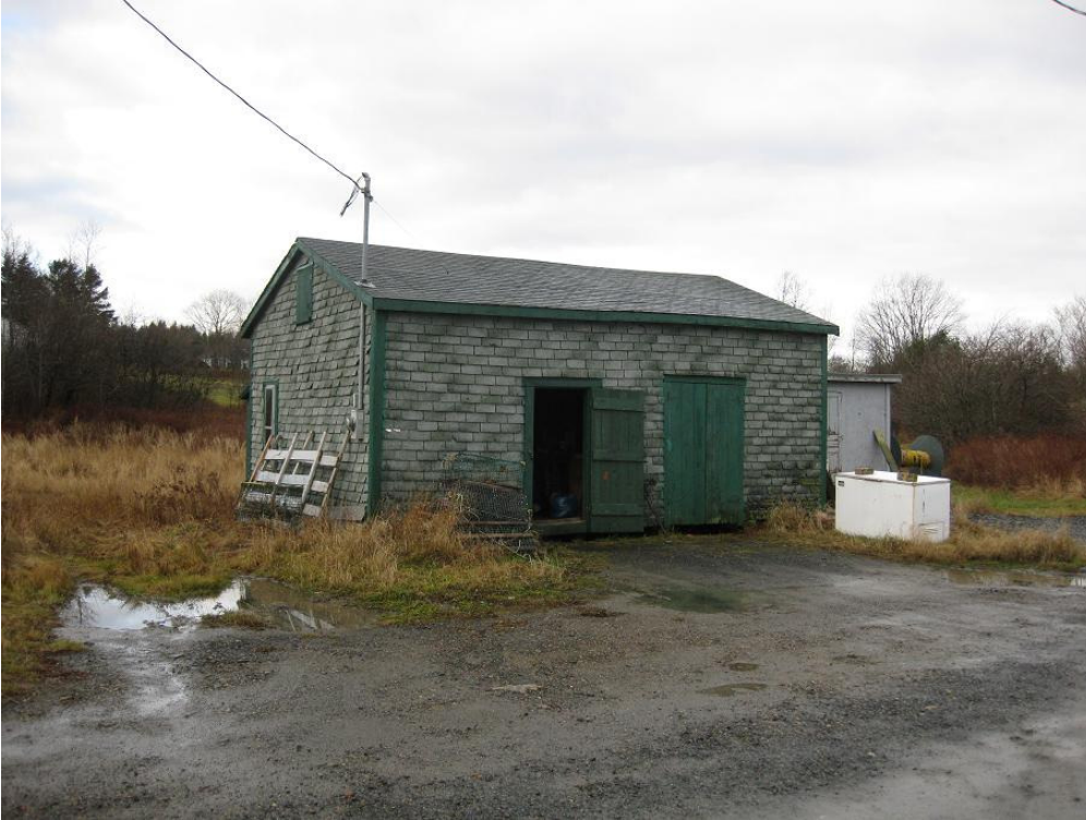
Figure 22 Bay Port fish shack after Hurricane Juan Sept. 28-29, 2003.
