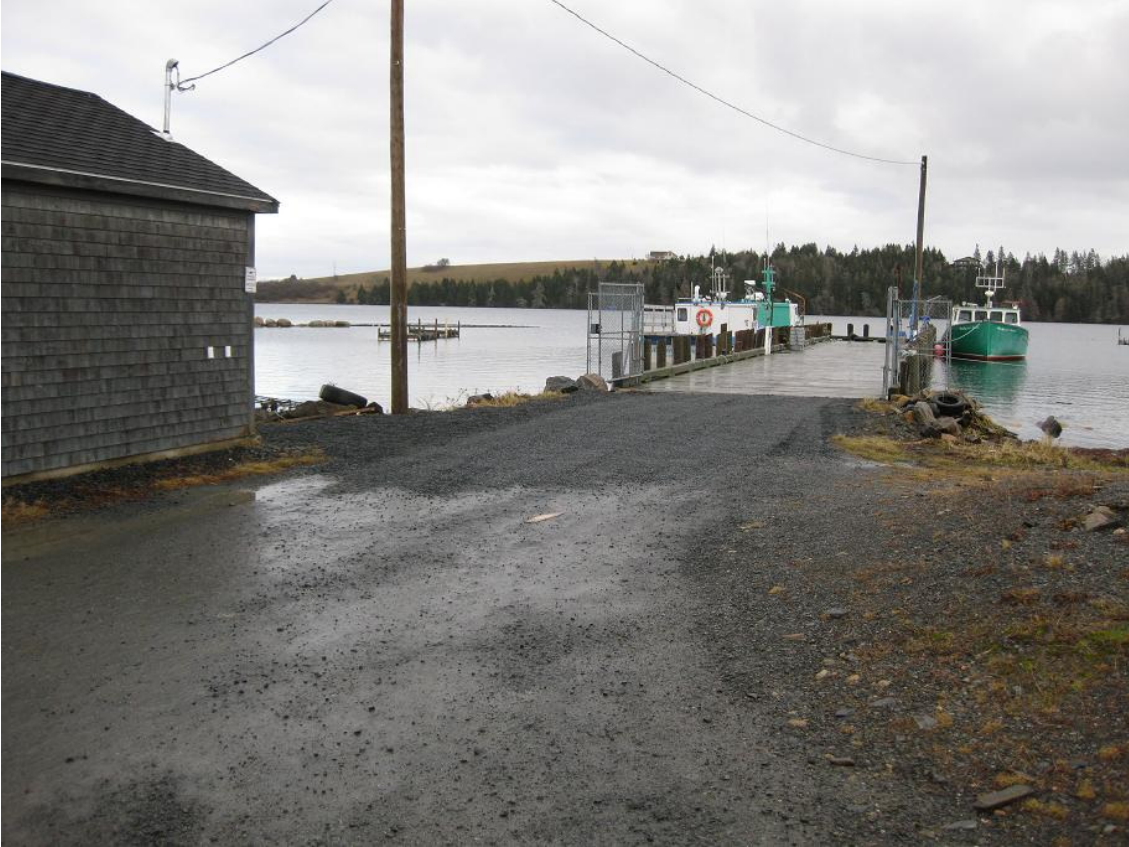
Figure 16 Bay Port wharf after Dec 6, 2010 storm surge. Nail in power pole marking the high-water elevation.
